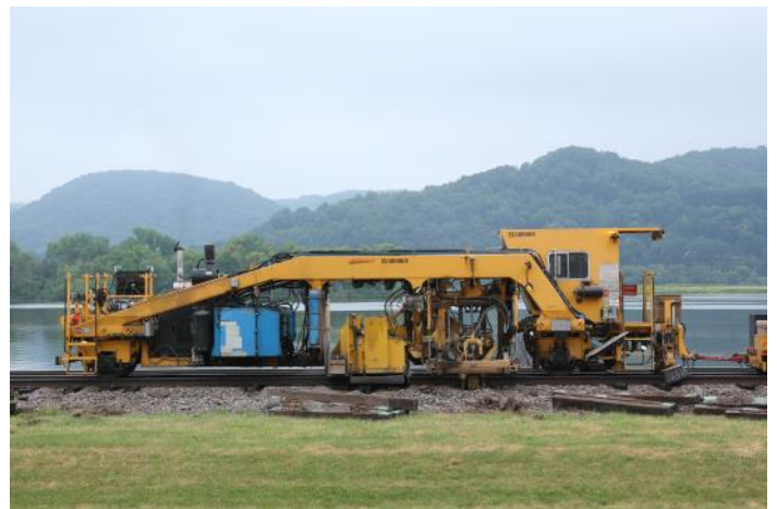
This is a multi-purpose tie aligning machine. The first unit, at left (obscured by shrouding), is a ballast broom. If any fine tuning of the tie placement is necessary, the second unit on this machine accomplishes that. Finally, a rotating broom brushes any ballast off the tie ends.
