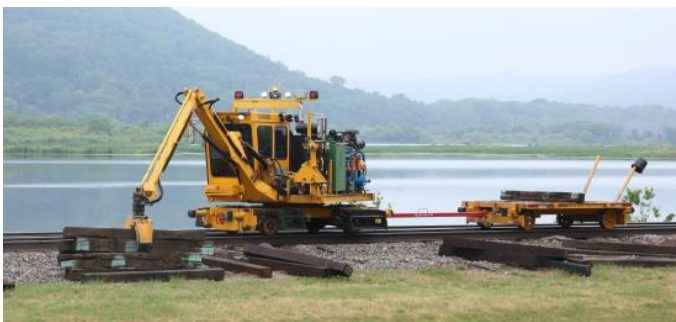
A tie handling crane removes the old ties off the roadbed
