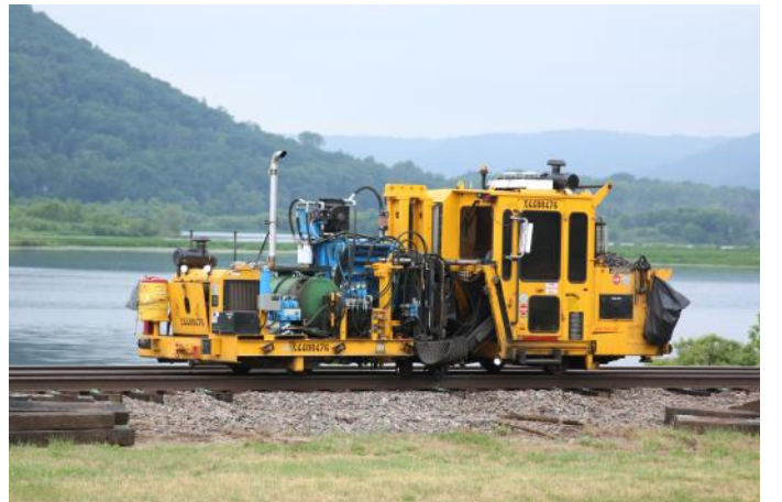
The spiker fastens the tie to the rail. Spike drivers are generally equipped with mechanical arms to shift the rail into proper gauge and hold it when inserting the spikes.
